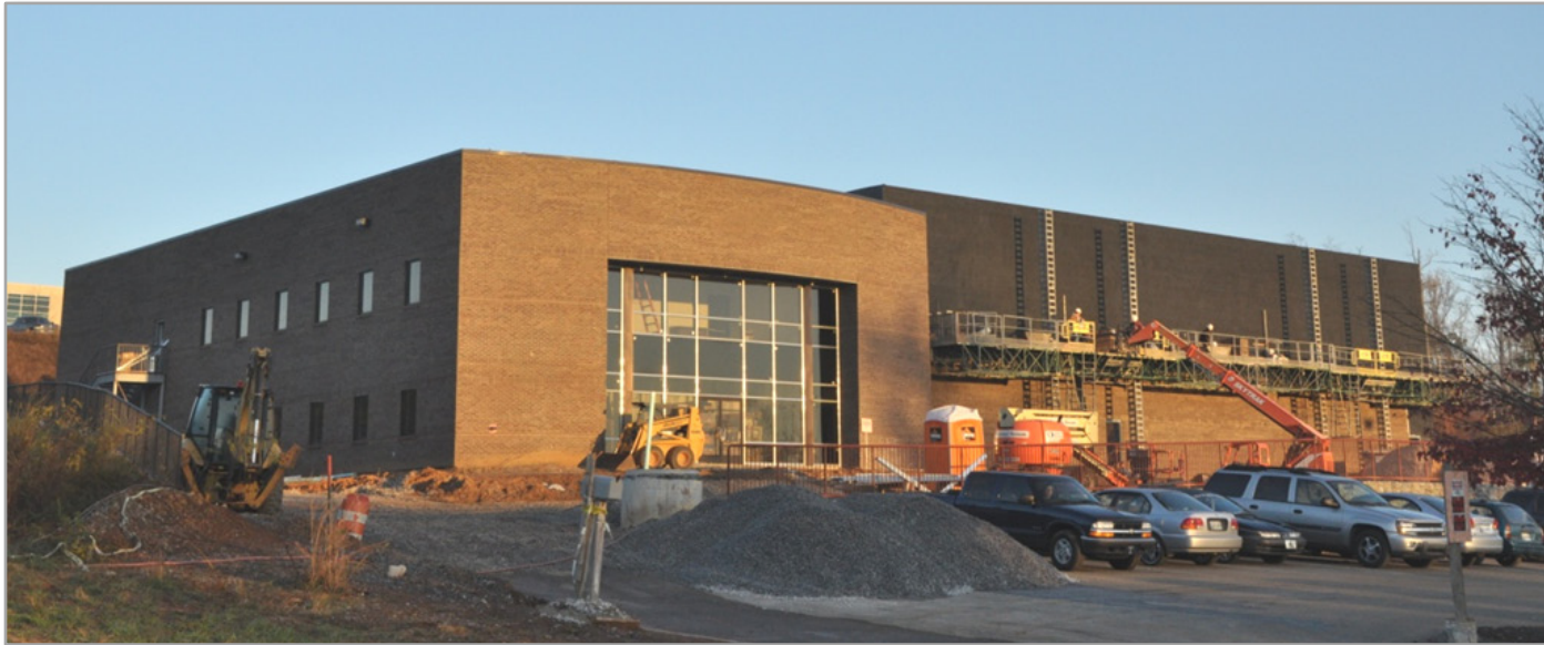
VSI laboratory construction status as of 11/11/2010
